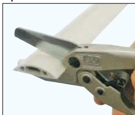
Cutting of cable protector
